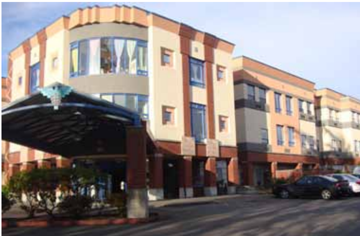
Figure 8. Sea Mar Community Health Centers, Administration Office
