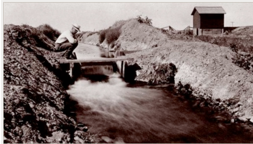
Figure 11. A lateral canal on the Garland Division of the Shoshone Irrigation District near Powell, 1913 (Homesteader Museum photo)
